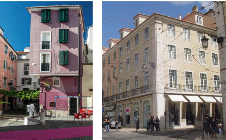
Fig. 2. Unreinforced masonry buildings in the Lisbon Metropolitan Area: ‘Pre-Pombalino’ buildings (on the left) and ‘Pombalino’ buildings (on the right).
