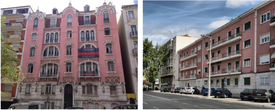
Fig. 3. Unreinforced masonry buildings in the Lisbon Metropolitan Area: ‘Gaioleiro’ buildings (on the left) and ‘Placa’ buildings (on the right).
